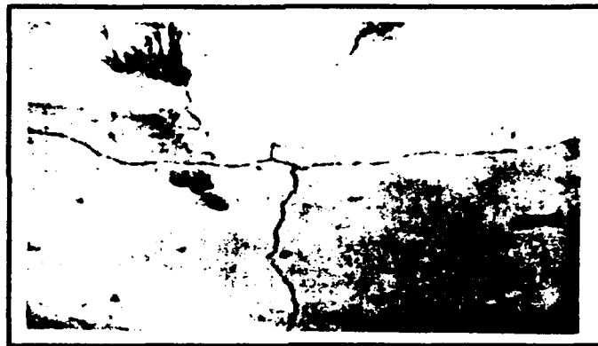
Figure 2.8 Typical drying shrinkage cracks (Reference 3)
